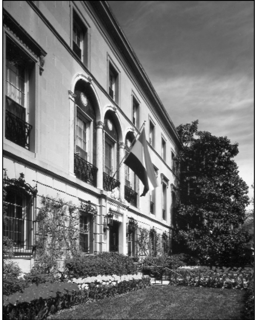
Officially known as the Royal Netherlands Embassy, the "Dutch Embassy" found McQuay Water Source Heat Pumps filled their sound and aesthetic needs perfectly.
