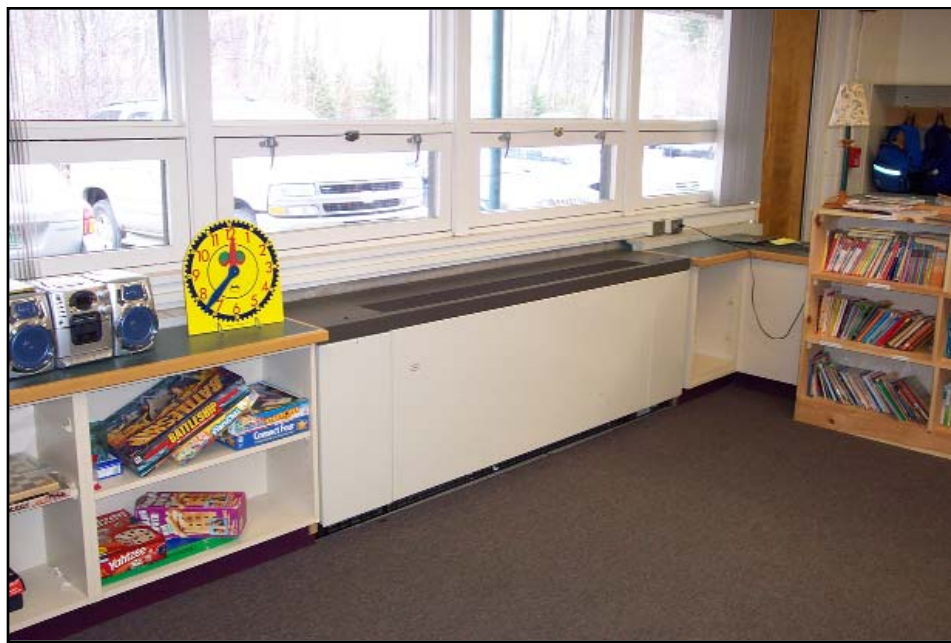
Flip-up panels on top of the new unit ventilators and easy-to-remove access panels on the front make maintenance easy and quick.
