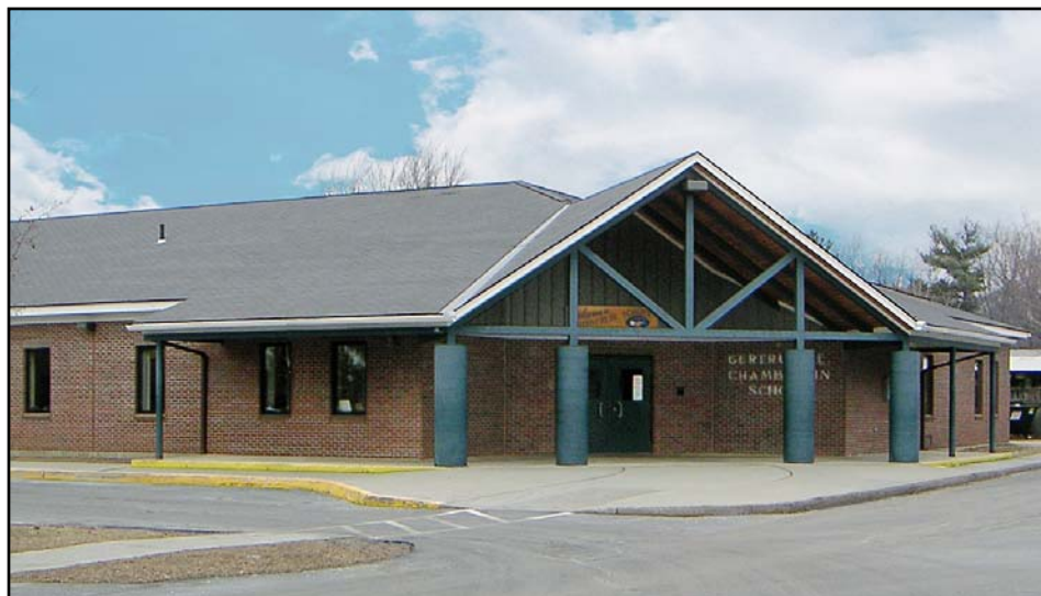
Installation of new unit ventilators at Chamberlin Elementary completes a renovation project begun in 1995. It included adding two new wings to the school as well as a district-wide heating renovation.
