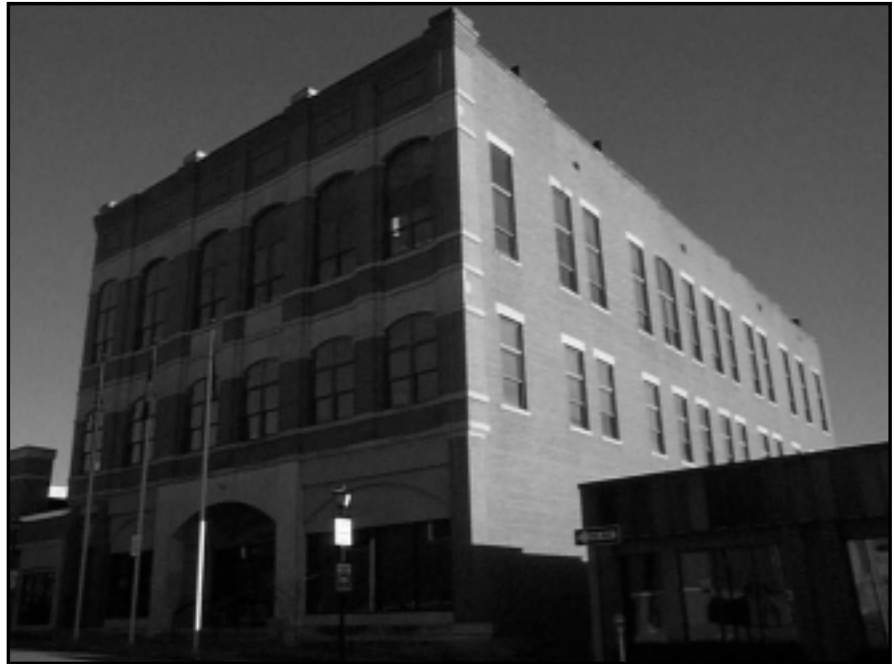
The Fayetteville City Hall is one of a collection of picturesque brick buildings situated in the historic town square. Maintaining its original historic character, while providing modern, efficient air conditioning, was a primary reason for selecting a McQuay SWT vertical self-contained system.
