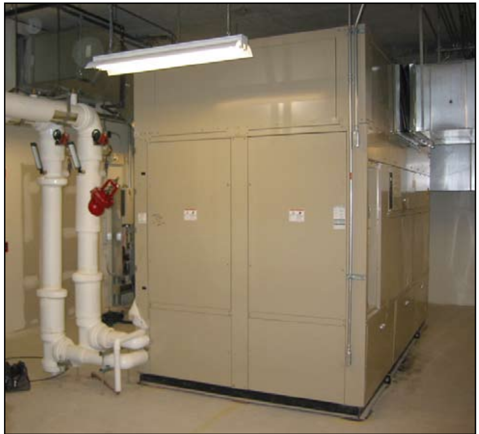
McQuay self-contained units can lower installed cost by $1.00 to $2.50 per square foot over chilled water systems. That's because they eliminate the need for large chiller equipment rooms and the additional pumps and chilled water piping that a central system requires.
