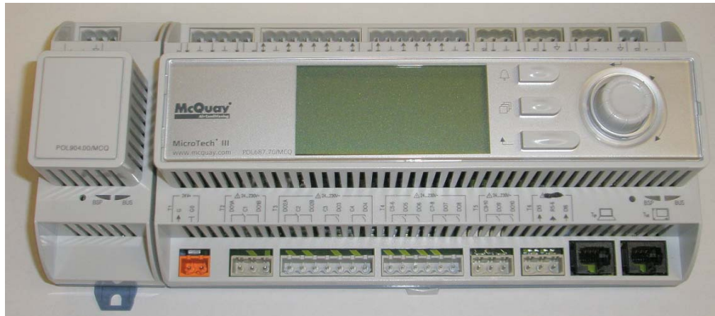
Figure 1. BACnet MS/TP Communication Module Attached to the Unit Controller
