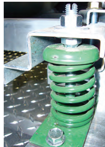
Figure 8: Spring Isolation
